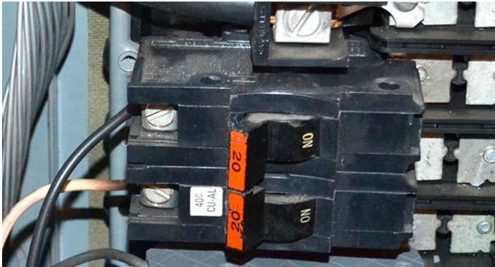
This is a close up view of a 20 ampere double-pole Stab-Lok breaker showing the handle shape and color.
